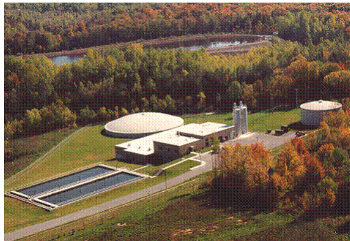
Hinckley Water Treatment Plant, circa 2000.
