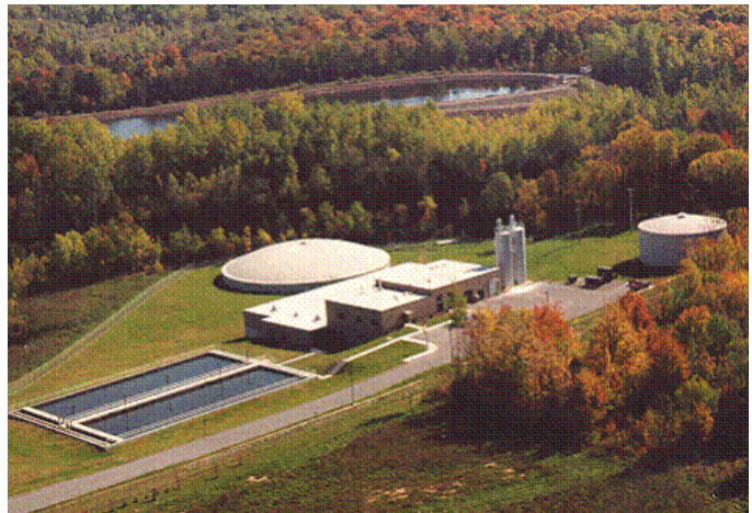
Hinckley Water Treatment Plant, circa 2000.
