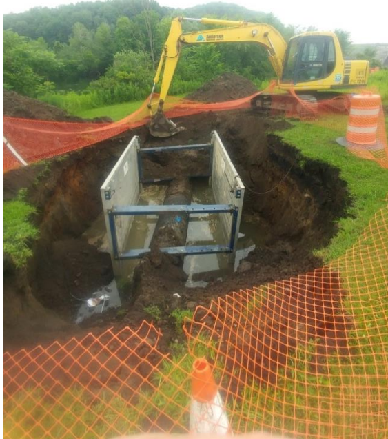
Preparing main for 36" linestop sleeve.
