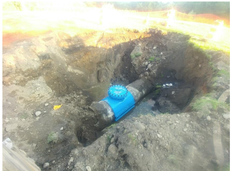
Sleeve ready for concrete foundation.
