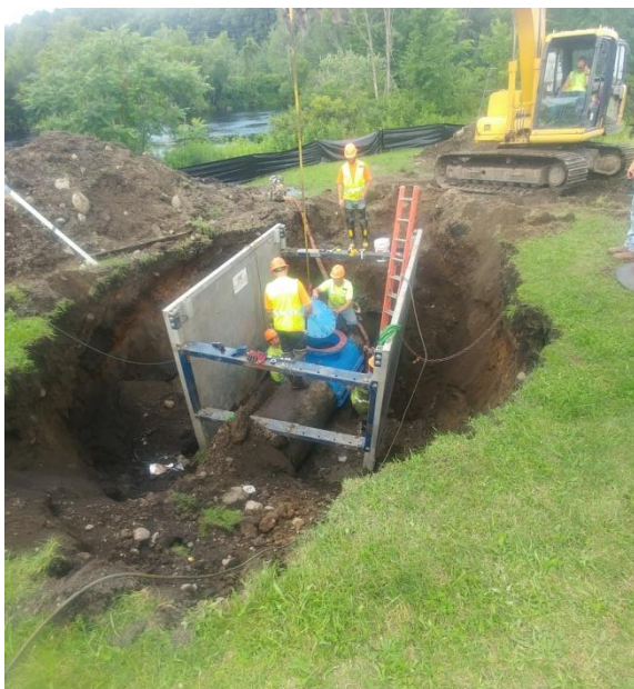
Installing linestop sleeve.
