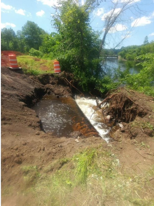
15 million gallons per day leak called in on July 4 th . Located and confirmed on 36" main at midnight.
