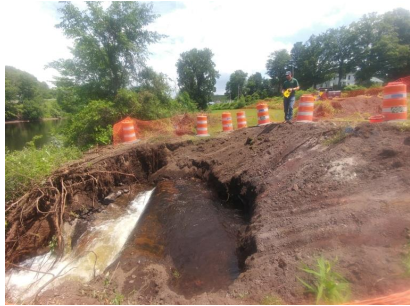
15 million gallons per day leak called in on July 4 th . Located and confirmed on 36" main at midnight.
