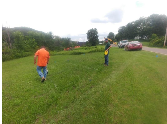
Laying out temporary valve locations and temporary bypass piping.
