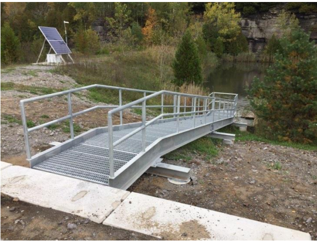
Solar Powered SCADA Monitoring System in background by MVWA.
