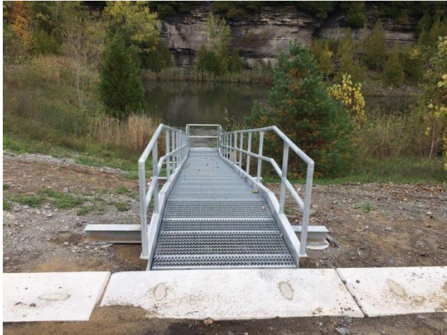
Ramp & SPEDES Sampling Station at Decant Lagoon.
