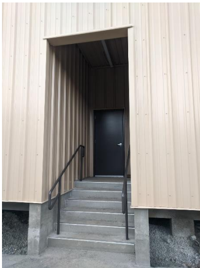
New steps and man door.
