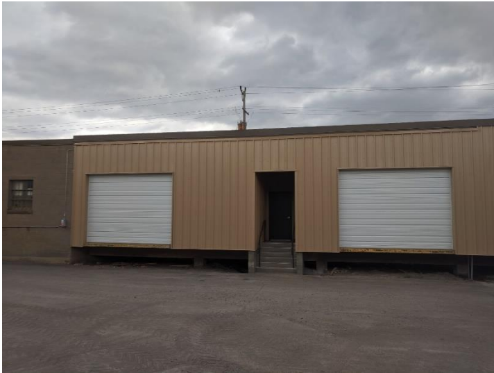
New Powered Overhead Doors for Material Access.
