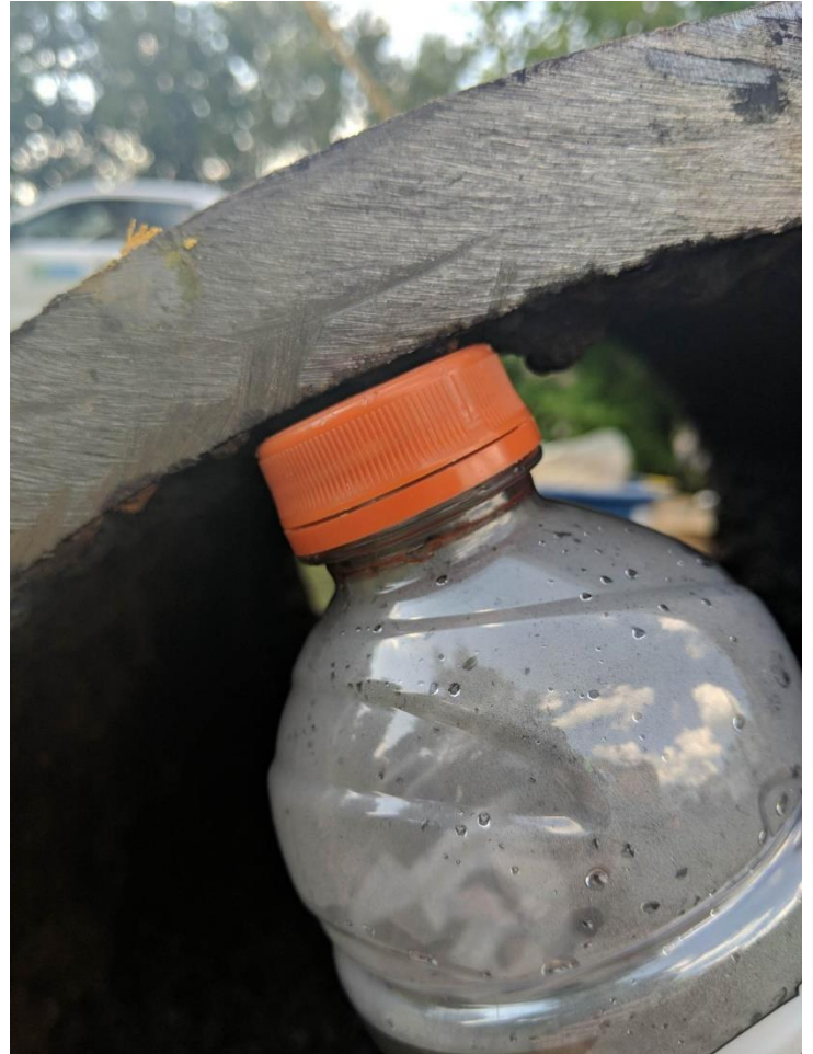
100-Year-Old 24" Cast Iron Pipe.
