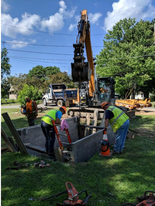
Safety Shoring at Work Area.
