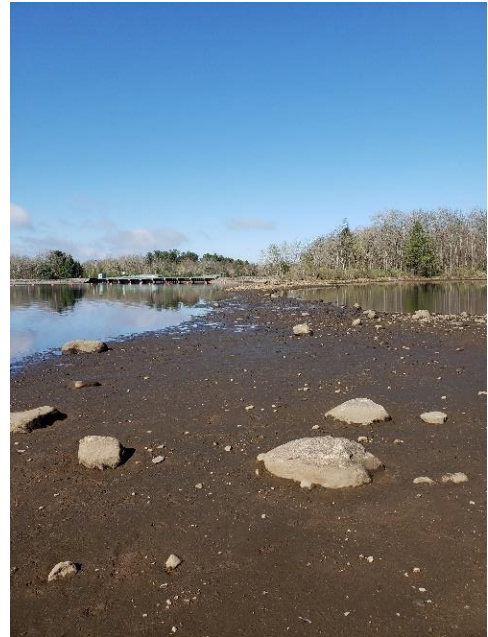
Transmission Main Route Approaching Prospect Dam. Main will go around Dam to the right.
