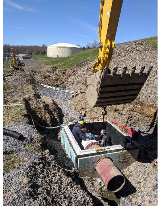
Setting new Magnetic Meter Assembly in Concrete Chamber.
