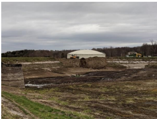
Placing cut material inside the Reservoir.
