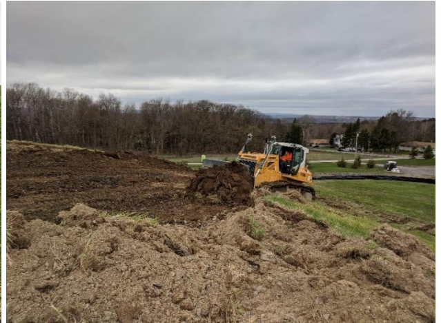
Cutting the Reservoir Embankment. Note Erosion Control Fabric.
