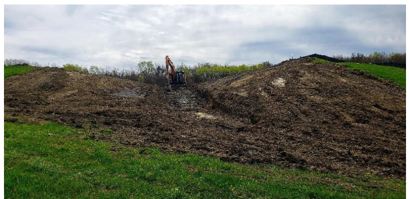
Near final elevation of new embankment grading.
